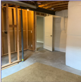
The Basement View
