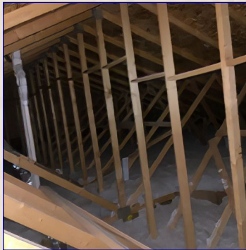
The Attic View
