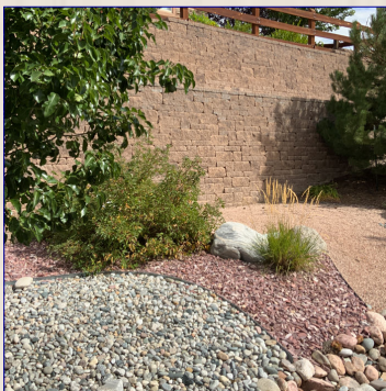
The Retaining Wall View
