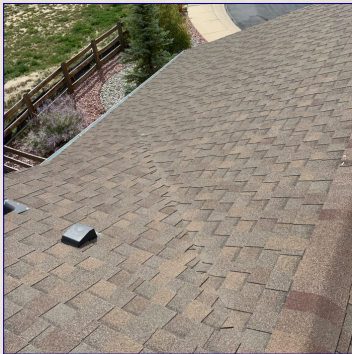
The Roof View
