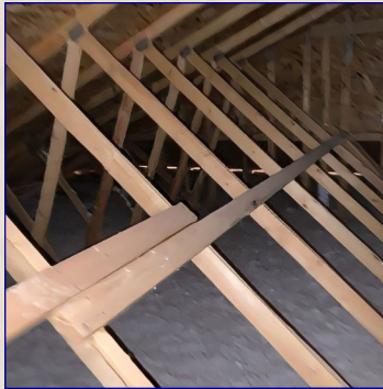
The Attic View
