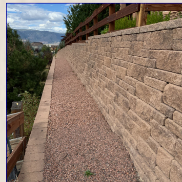
The Retaining Wall View
