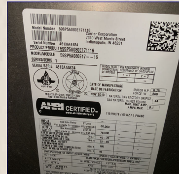
The furnace, data tag
