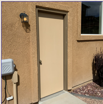
Garage exterior service door view.
