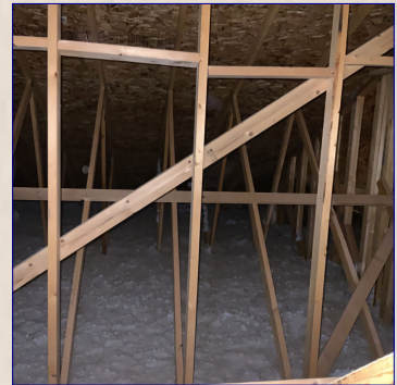
The Attic View
