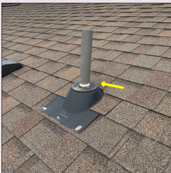
The Plumbing Vent(s)
