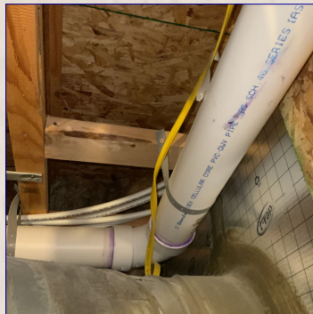
The visible drain/waste piping.
