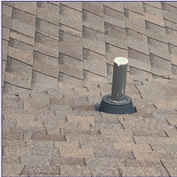
The Plumbing Vent(s)
