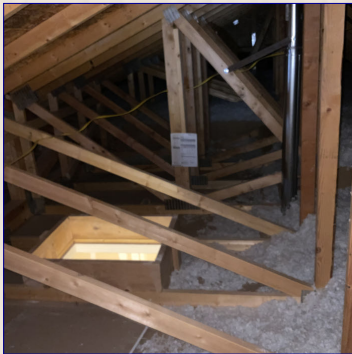
The Attic View
