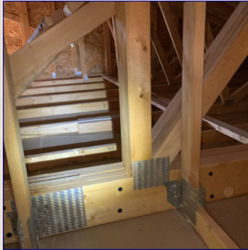
The Attic View
