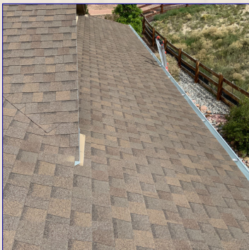
The Roof View
