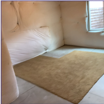
The Basement View
