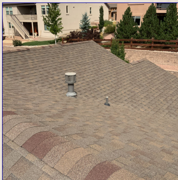
The Roof View
