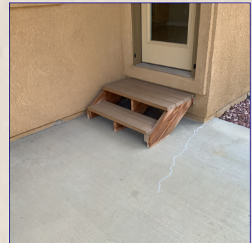
The Steps/Stoop View
