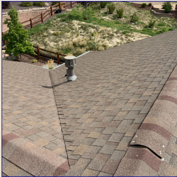
The Roof View
