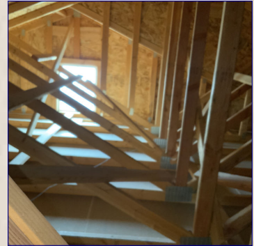
The Attic View
