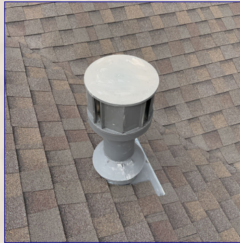
The Chimney Chase
