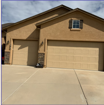
Garage overhead door view.
