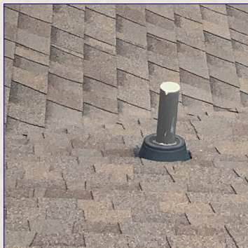
The Plumbing Vent(s)
