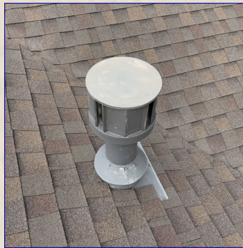
The Chimney Chase
