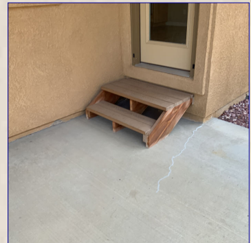
The Steps/Stoop View
