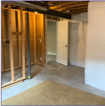
The Basement View
