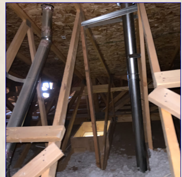
The Attic View
