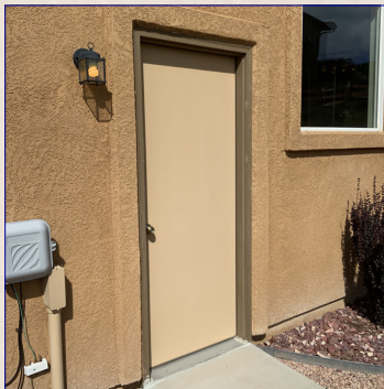
Garage exterior service door view.
