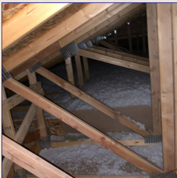
The Attic View
