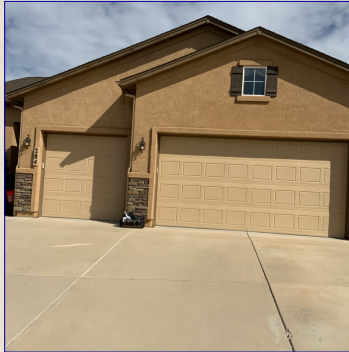
Garage overhead door view.
