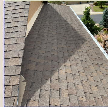
The Roof View
