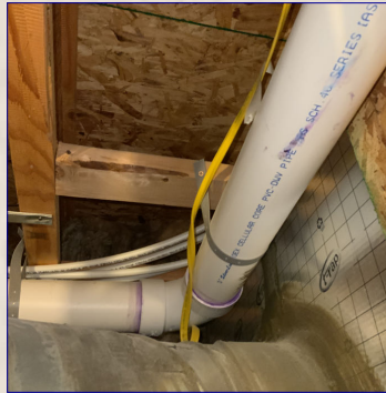
The visible drain/waste piping.
