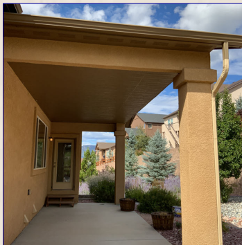
The Deck/Porch/Patio Cover View
