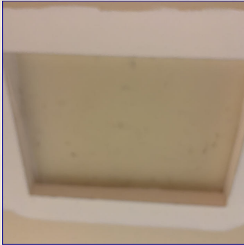
The Attic Access View
