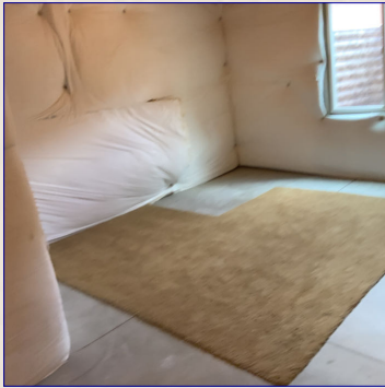
The Basement View
