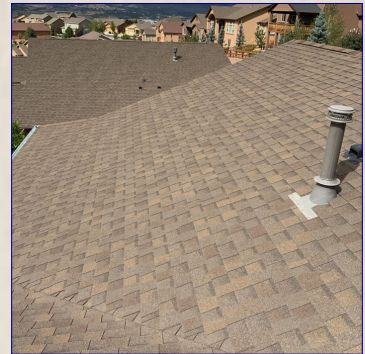
The Roof View
