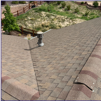
The Roof View
