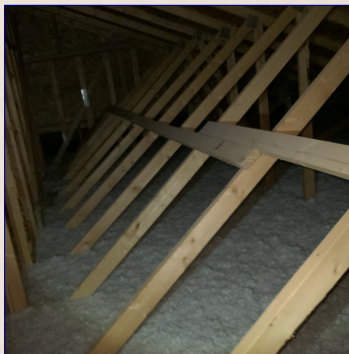
The Attic View
