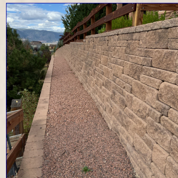
The Retaining Wall View
